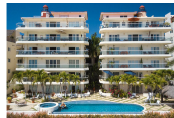
Faro Real #1 Tower Two 104 Calle Hidalgo Punta de Mita Nayarit, Mexico
